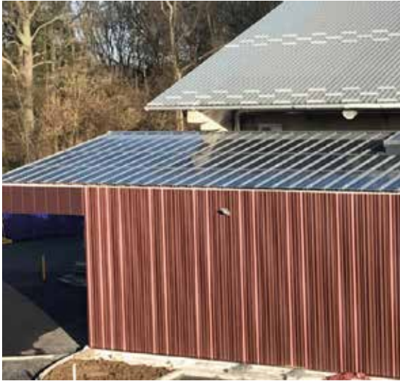
Pilot installation of thin film PV solar cells on roof new CRM building
